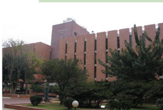
香港理工大學包玉剛圖書館安裝了蒸發式冷卻塔 Hong Kong Polytechnic University Pao Yue Kong Library Building is now equipped with evaporative cooling towers
